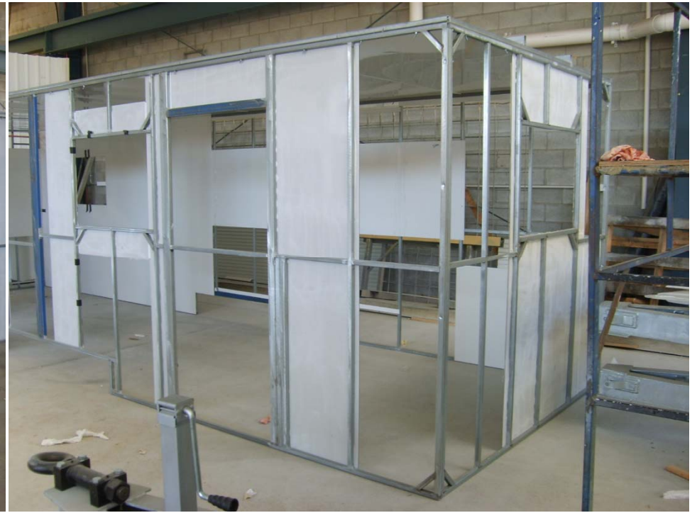
Construction of walls of one Mobile Training Unit
